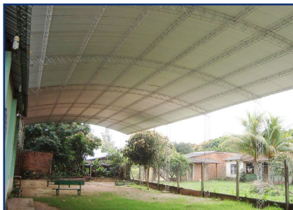
The church roof is now completed in Bolivia
