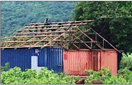
Construction of our “outdoor classroom” at the Nsanga Agriculture Training Center
