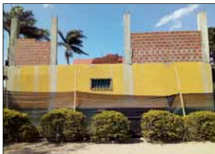
The walls of CENTEB going up
