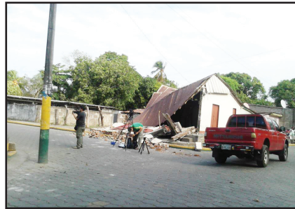
Damage to a building in Nagarote, Nicaragua
