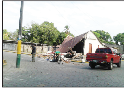
Damage to a building in Nagarote, Nicaragua
