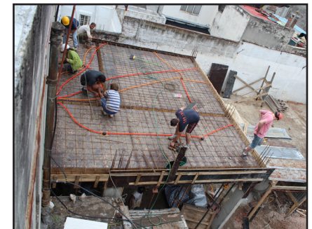
Construction at Grace Bible Church Montevideo, Uruguay
