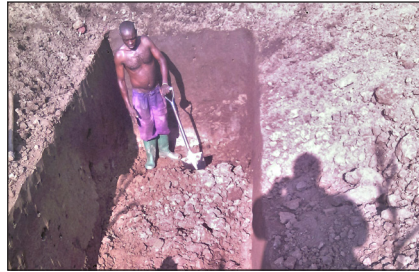
Construction at the primary school in Tanzania
