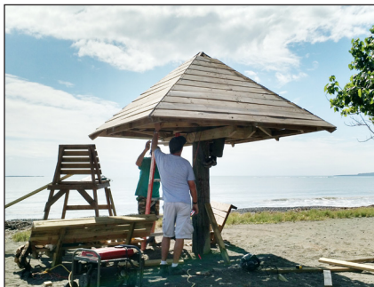
Members of the team repairing the fallen gazebo
