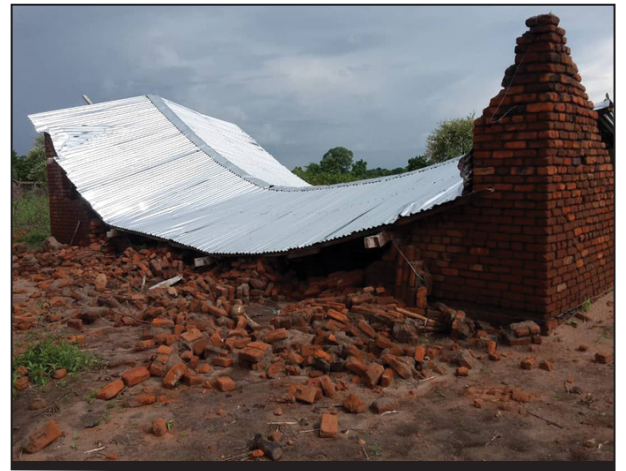
Damage from Cyclone Ana
