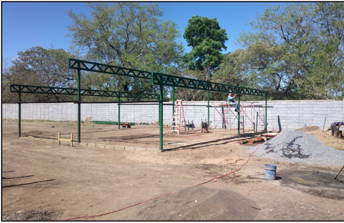
Construction of the first building on the property in Nicaragua
