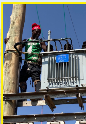
Dulla, from Tanesco hooking up an electrical transformer at our plateau property. First time to have electricity that is not solar or generator powered! Hurray!
