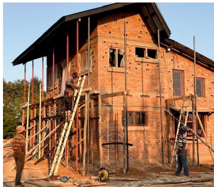
Construction on the apartment above our pottery studio.
