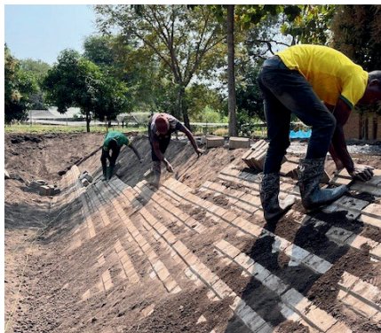
Building up the walls of our new fish pond utilizing interlocking compression bricks we made from soil and cement.
