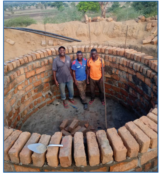
Jericho, Bandanga, and Martin in the “step down” water collection tank of the Lyanza water project. This project has brought water to a primary school, village market place, and one of our AG venues.
