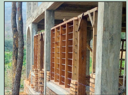
Masonry work going on as we fill in between the poured concrete columns. It is our hope to move into this home before Christmas.
