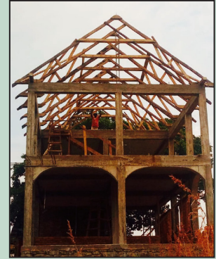
The trusses went up on our training/team house at our Nsanga village AG center last week.
