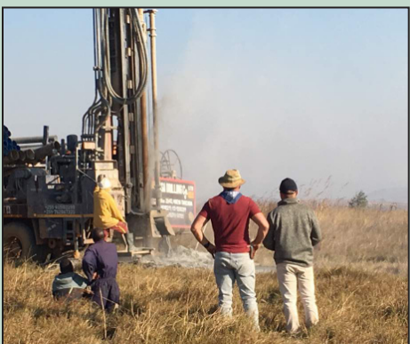
Well drillers at the plateau tree nursery.
