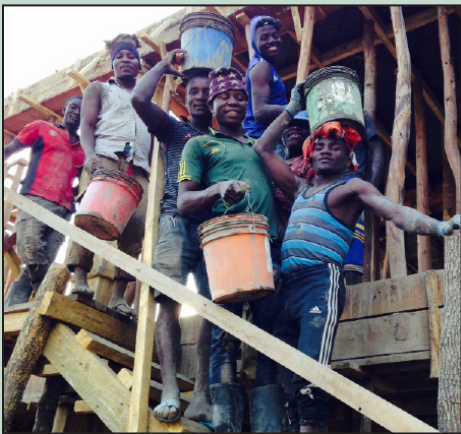
Most things are still done by hand where we live. It is effective and allows us to hire local men who love the salary they make while helping us. It is also one of the best ways to make relationships! These guys helped mix concrete and haul it by the bucket to build our home.
