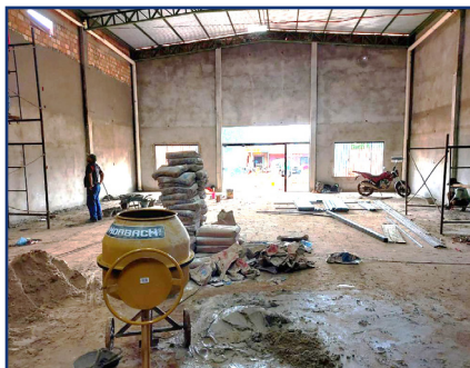
Paraguay church—before the remodeling project
