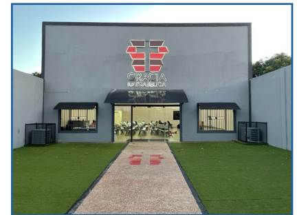
The finished exterior of the church
