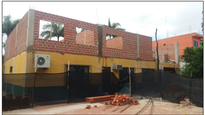
The construction of the Training Center should be complete by the end of the year
