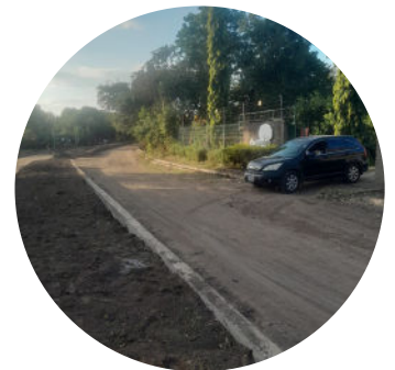
ROAD CONSTRUCTION AT THE CHURCH ENTRANCE
