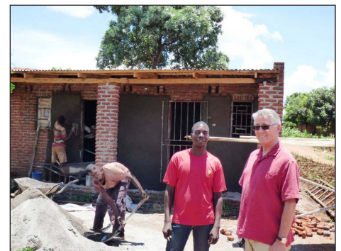
Bill and Yamikani were the supervisors of these building projects.
